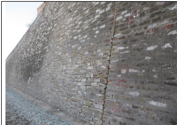
K33+610~K33+620 左侧挡护开裂
